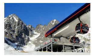
skiers to Skalnaté Lake in seven minutes and exceeds the vertical drop of 599 m. The cableway resists winds up to 22-24 m/s. The start station of the gondola Štart - Skalnaté Lake starts at 1,170 m a.s.l., and the end station is located at 1,772 m a.s.l. The all-year most attractive cableway is still the elevated gondola to Lomnický štít which can get visitors to the top of the second highest peak of the High Tatras just in 8 minutes, and which has been in operation for 75 years now.
